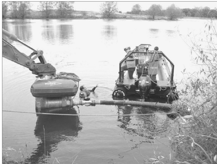
Figure 3. Launching of Submersible Pump and Flotation Unit
